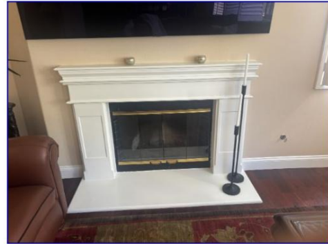
Gas line is capped and the fireplace is inoperable
