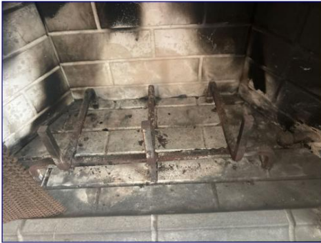
The Fireplace View: Gas pipe has a plug and the fireplace is unusable
