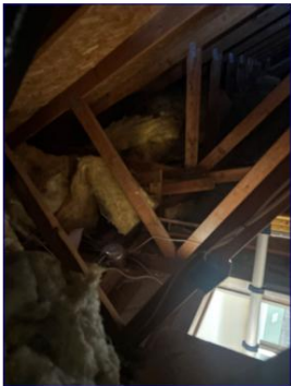
Scuttle Hole not insulated
