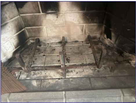
The Fireplace View: Gas pipe has a plug and the fireplace is unusable
