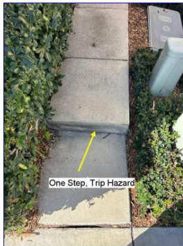
One step on the walkway is a trip hazard. Recommend a professional contractor to fix
