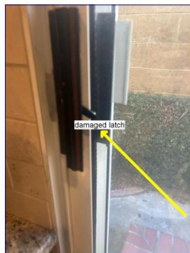
The door latch not working
