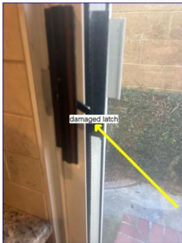
The door latch not working
