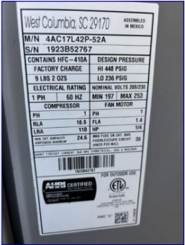
The air conditioner compressor/condenser data plate.
