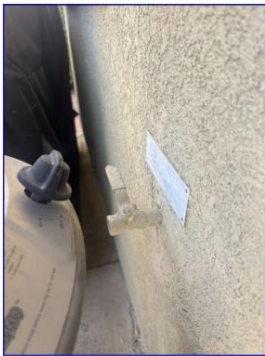
Unused gas outlet needs to be capped with a real plug on the Westside wall in the back patio
